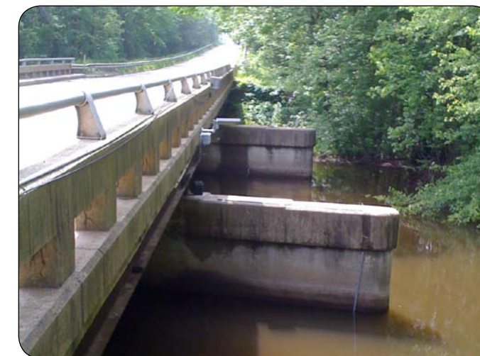
Bridge-mounted data logger.
