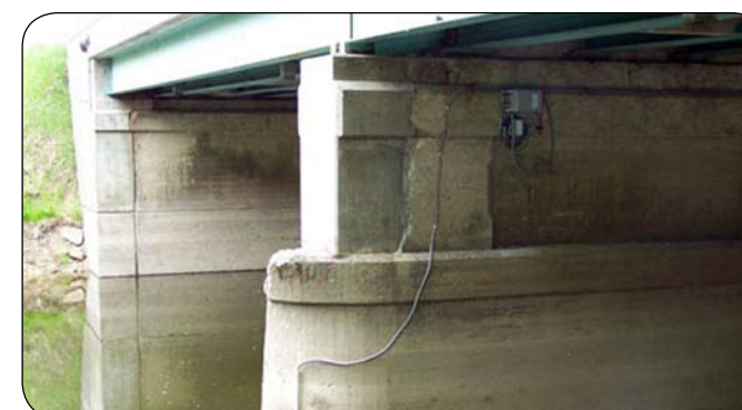
NexSens 3100-iSIC data logger with cellular telemetry.
