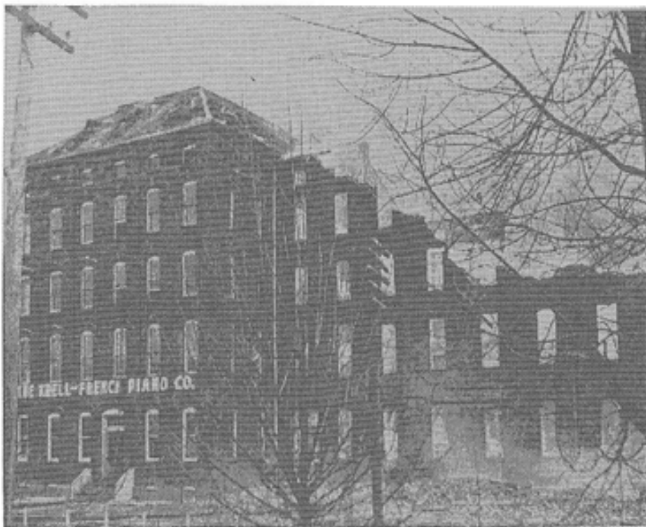
Damage to the Krell-French Piano Works.
