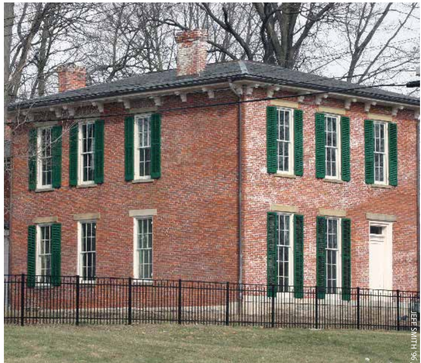
Exterior restoration work on the historic Geiger House has been completed.
